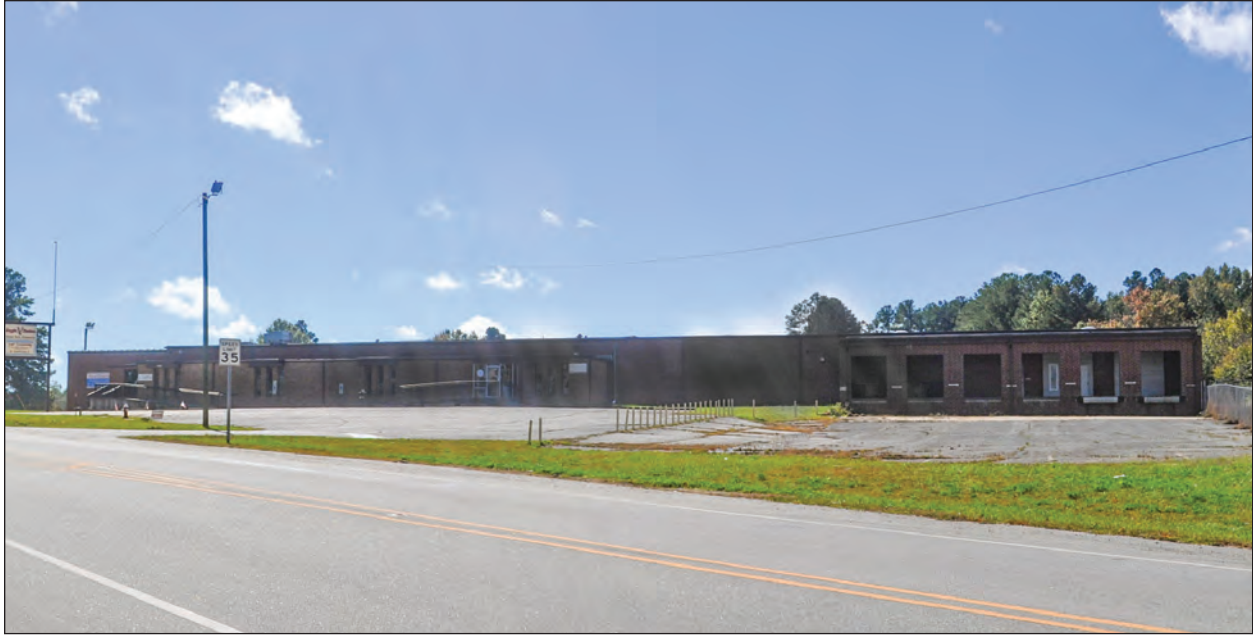
Figure 3.15. U.S. Industries Headquarters/Lampart Tables Factory
