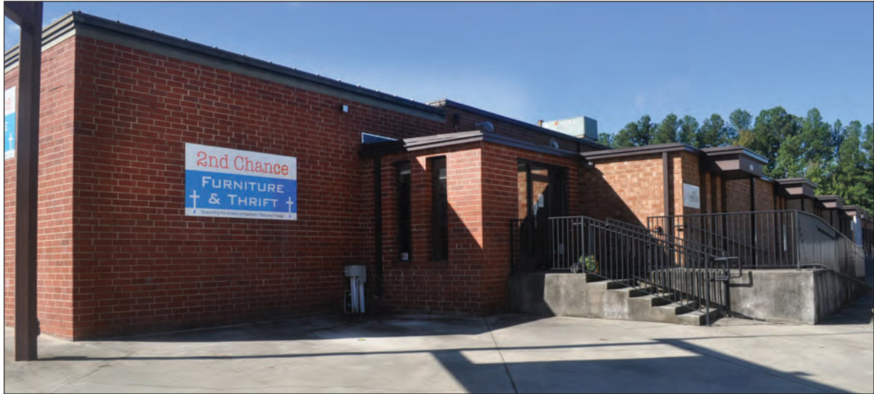
Figure 4.5. Northeast Corner Showing Office Section and Addition Entry
