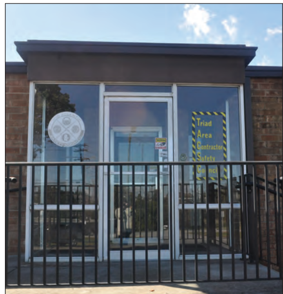
Figure 4.4. Glass Entry Door on North Side of Office Section
