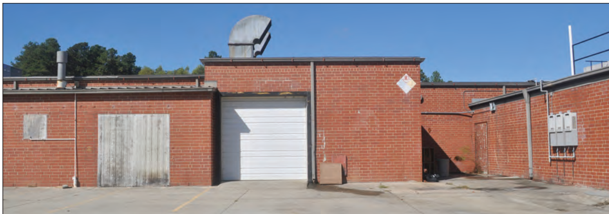
Figure 4.10. Small Additions to East Side of 1963 Building
