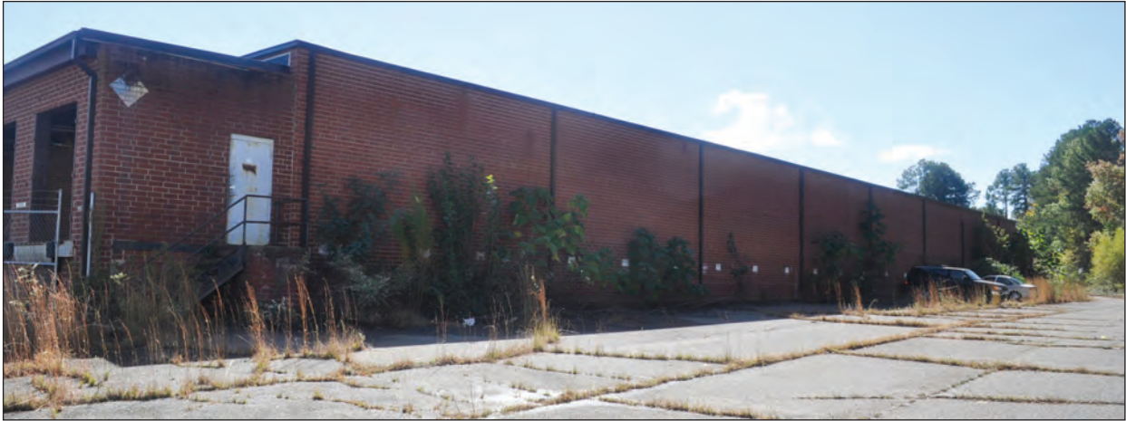
Figure 4.7. West Side of Shipping/Receiving Addition
